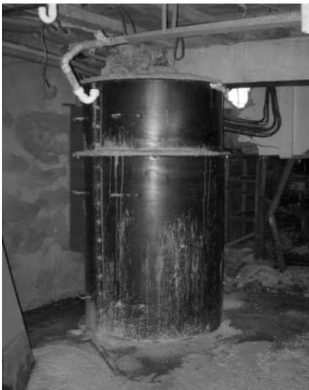
Damaged columns with completed encasement
