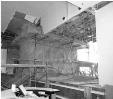
Overall View of Repair Using Shotcrete
