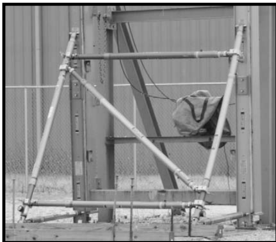
Photo of raker using strut bracing – no wood needed
